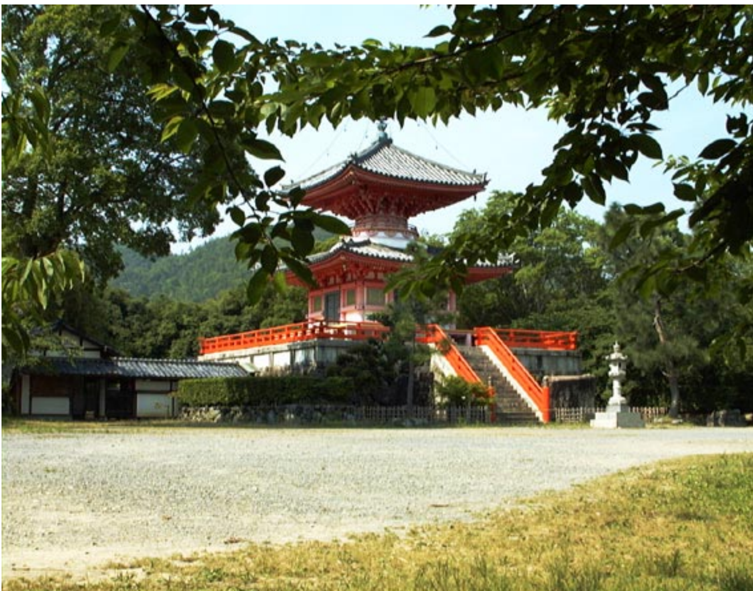
Tahoutou Building (1998.5.23) in the lakeside
