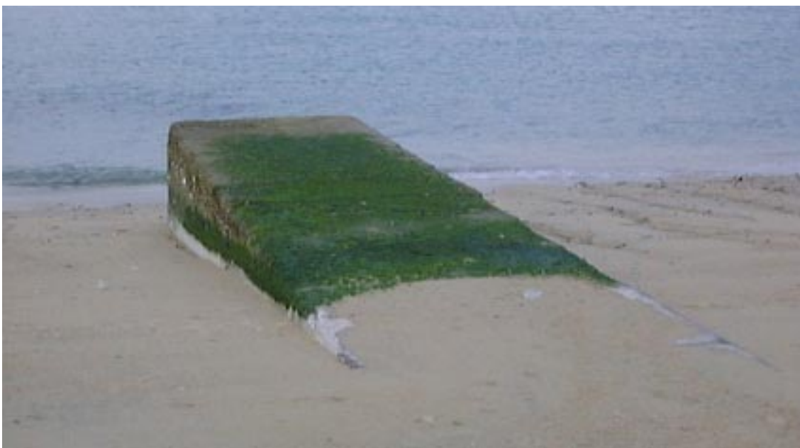
Watergate No.2(1998.3.13) now being exposed by the accelerated removal of sand layers
