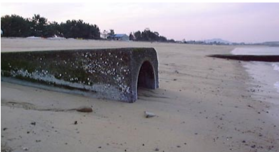
Front side of Watergate No.2 (1998.3.13) composed of a single Pipe
