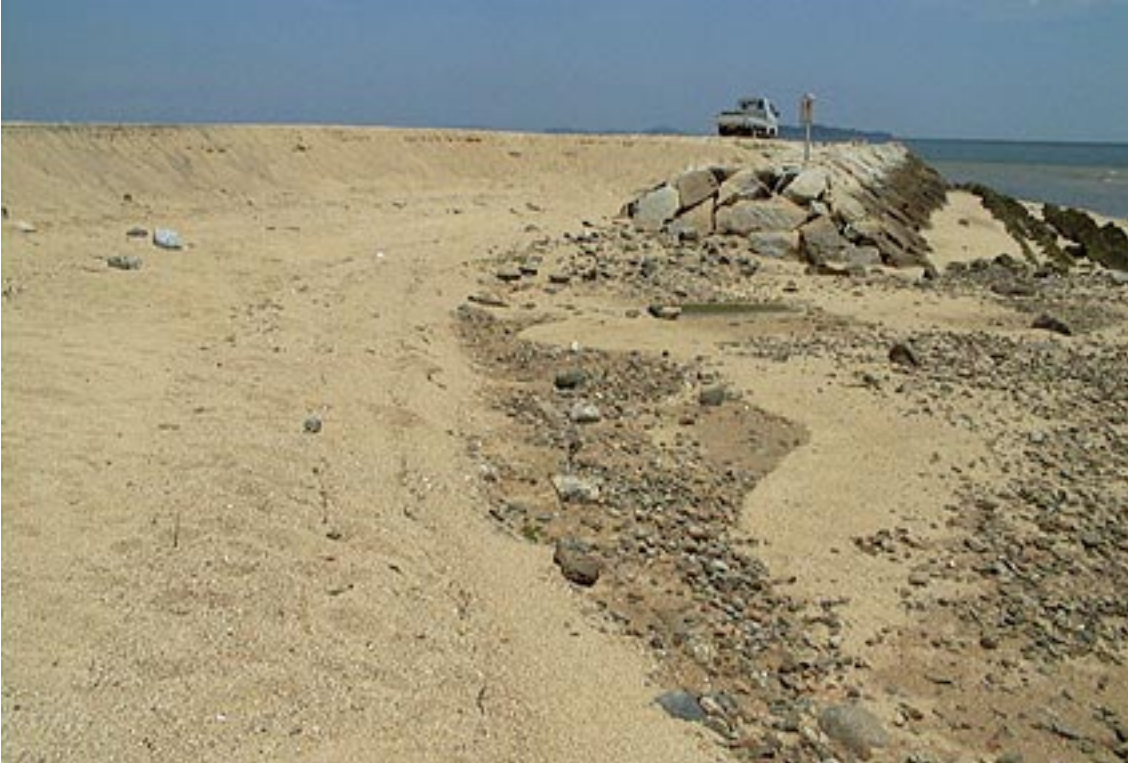
Massive Removal of Sand layers (1998.7.5) around the North Bank of River Tonda
