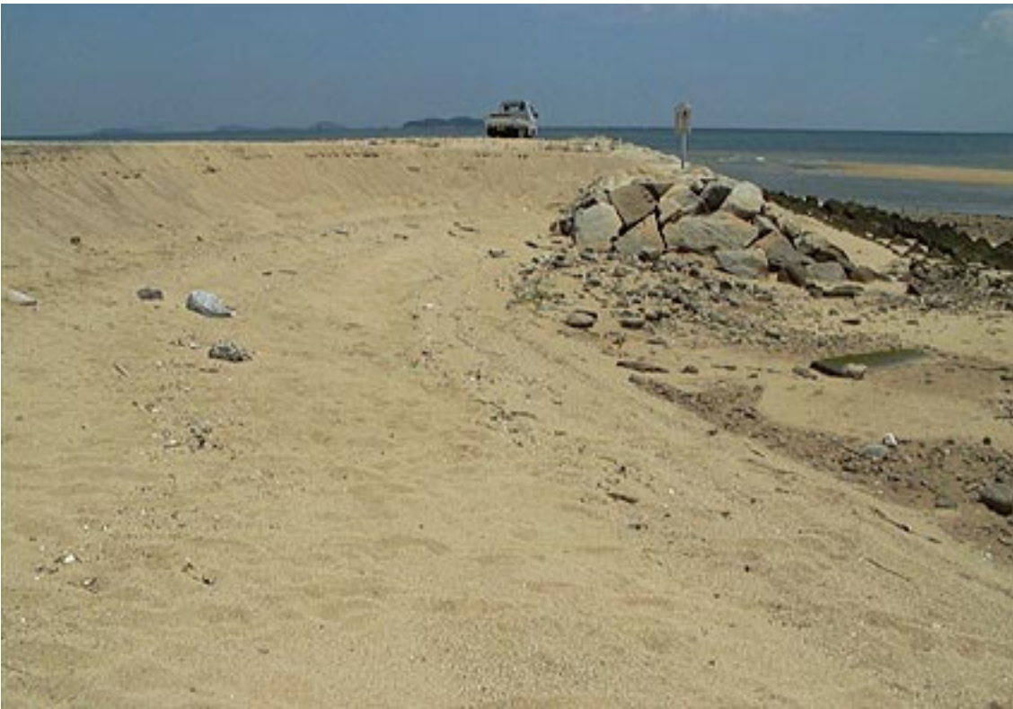
Also Massive Removal of Sand layers (1998.7.5) around the North Bank of River Tonda
