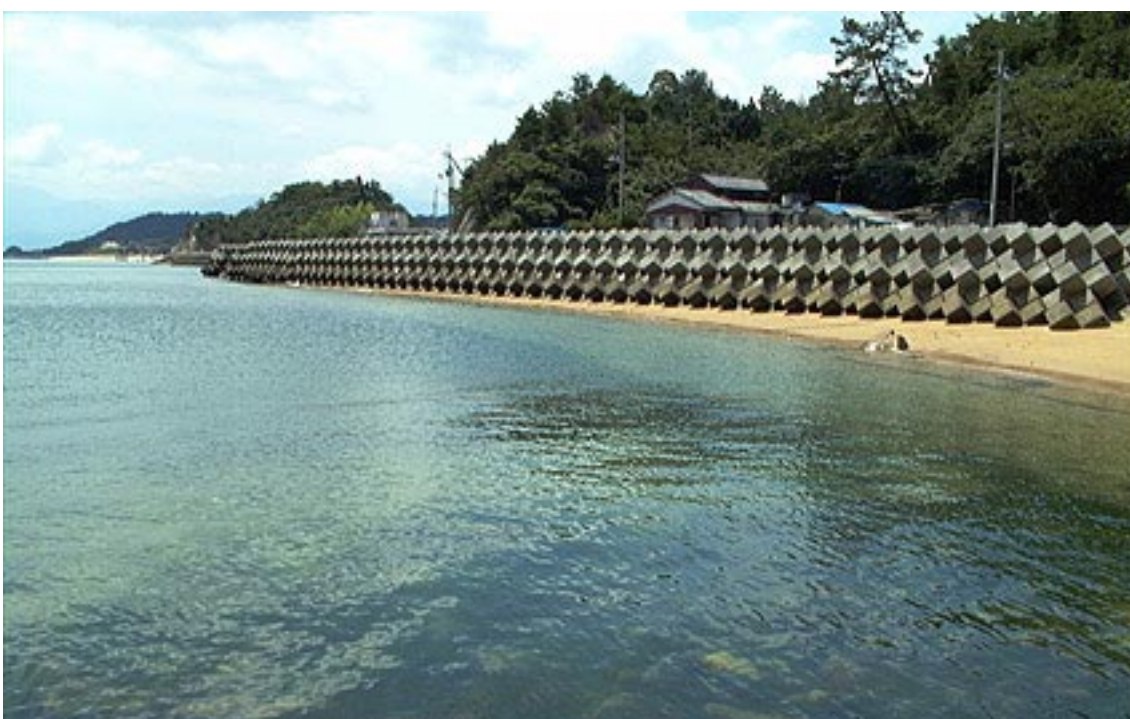
Block Wall in Okiura District (1998.7.5) showing the acceleration of removal of sand layers
