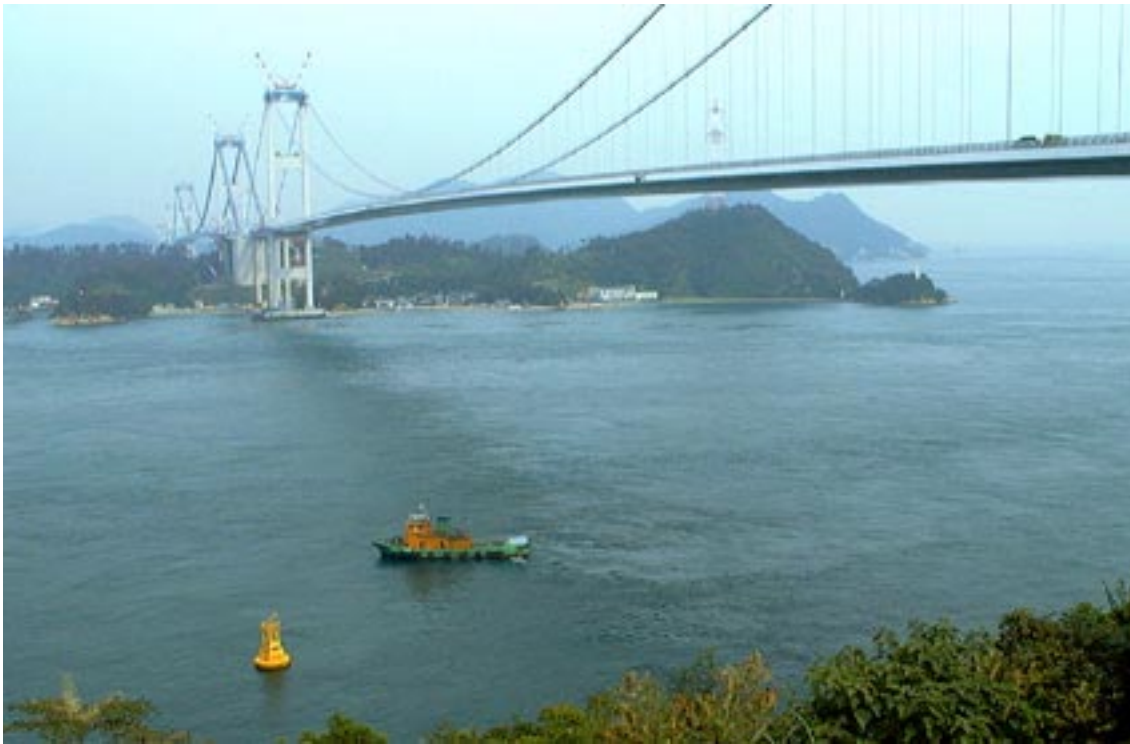
The Great Bridge(1998.10.10) crossing over the Kurushima Strait
