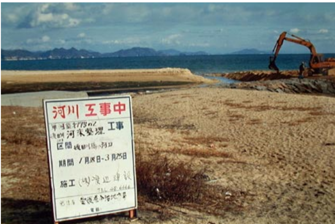
Cutting the Sand Bridge for making water exit into the Sea (1985.1.25) Three photos show the active power of sand accumulation in 10 years ago
