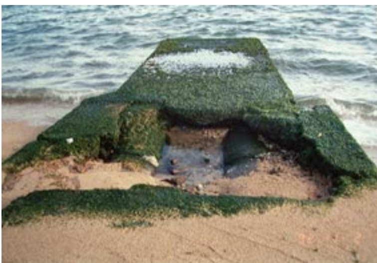
The Same Watergate in 1992.11.2 showing acceleration of decrease of Sand layer
