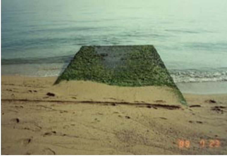
The Watergate of ODAGAHAMA in 1989.7.23 Note the level of Sand layer in both sides And it is higher in the left than in the right side
