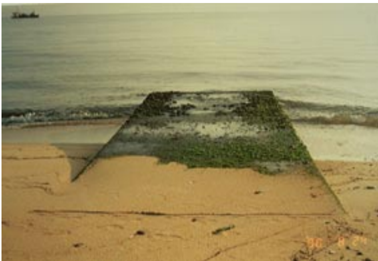
The Same Watergate in 1990.8.24 showing decrease of Sand layer in both sides
