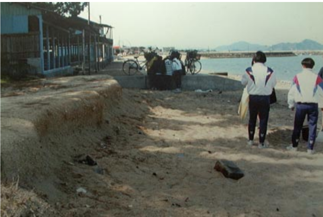
Massive Removal of Sand layers by Storm(1985 March) in SAKURAI Coast
