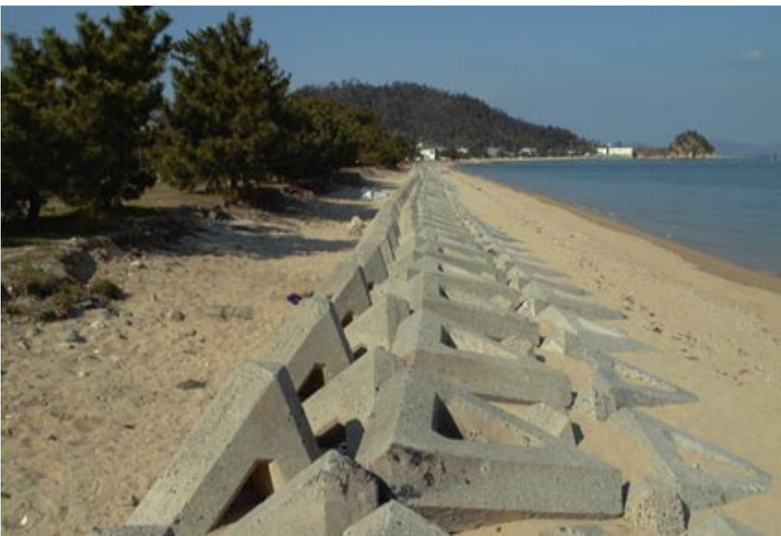
Block works in the Toragahana Coast neighbouring Ishifuro (1998.1.31) showing the wave in storm had easily come over the block line and will acceleate more removal of sand layers
