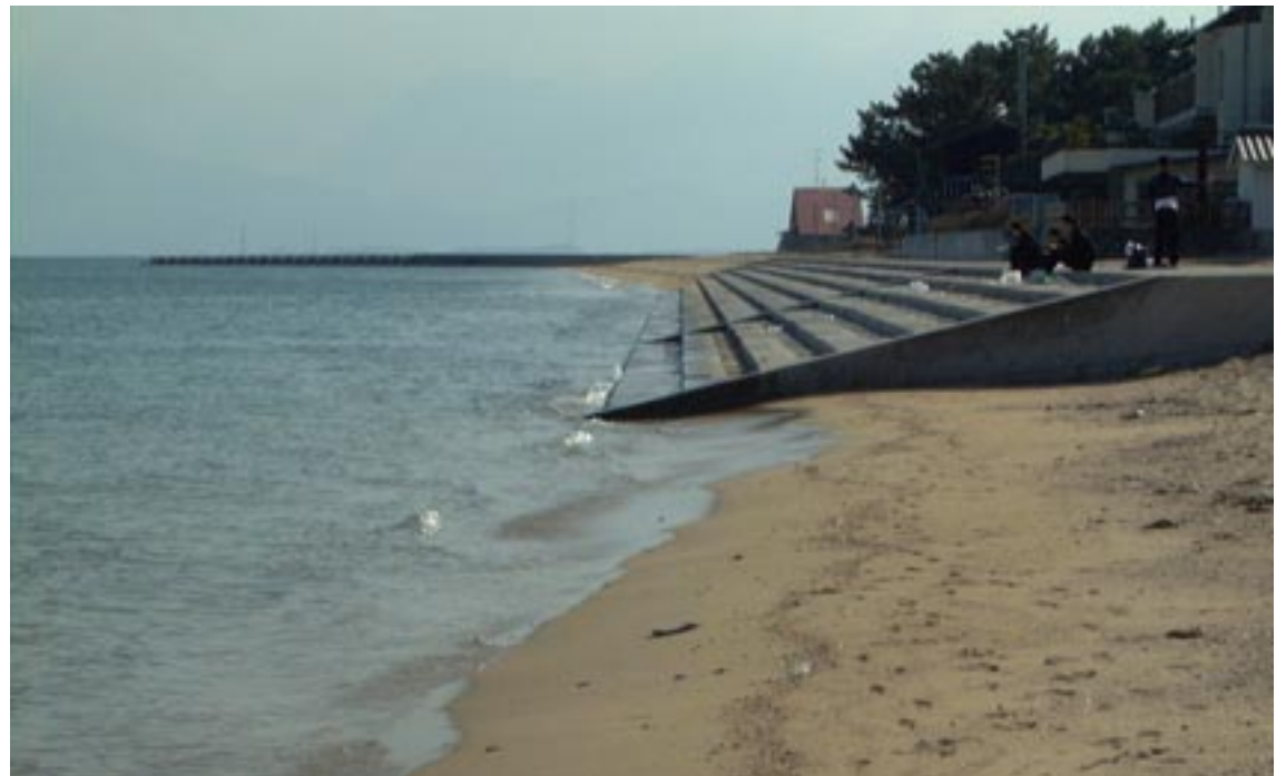
The Sea Water coming nearer to The Restaurant (1998.1.31) suggesting concrete step work might accelerate the removal of sand
