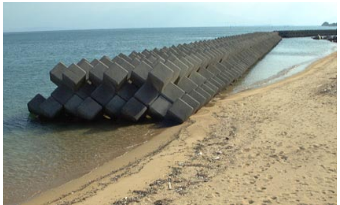
A Sample Photo verifying Block works accelerate the removal of sand (1998.1.31)
