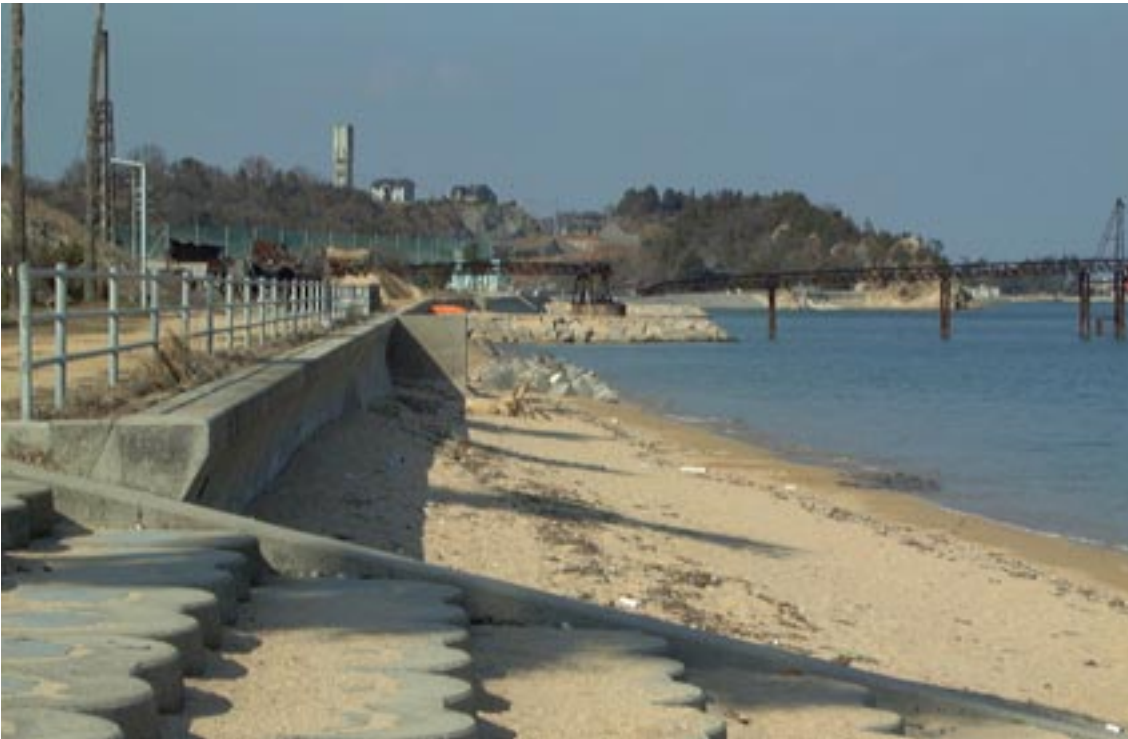
Block works of Okiura Coast (1998.1.31) showing active removal of sand layers
