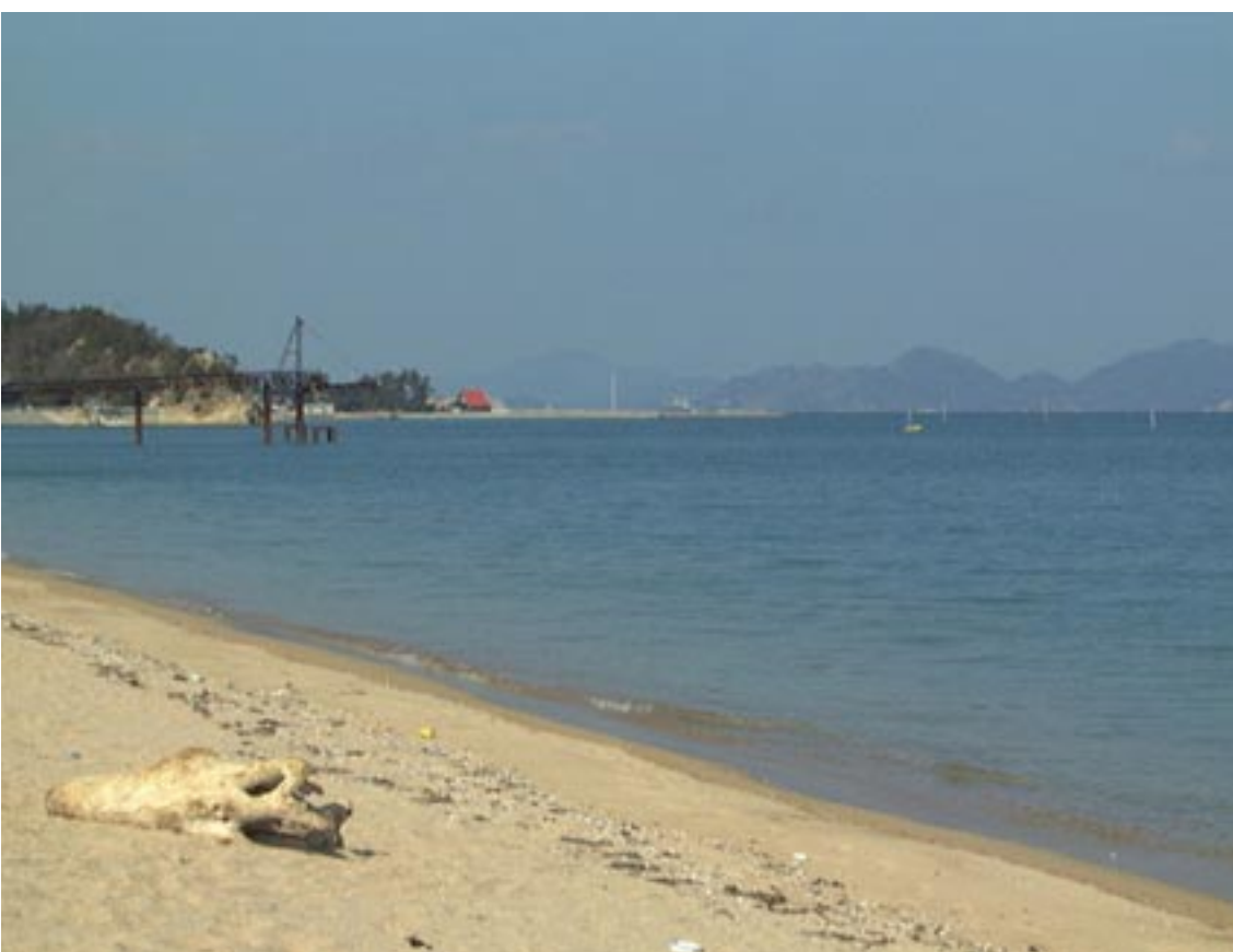
Far view of The Great Bridge (1998.1.31) from the Okiura Coast
