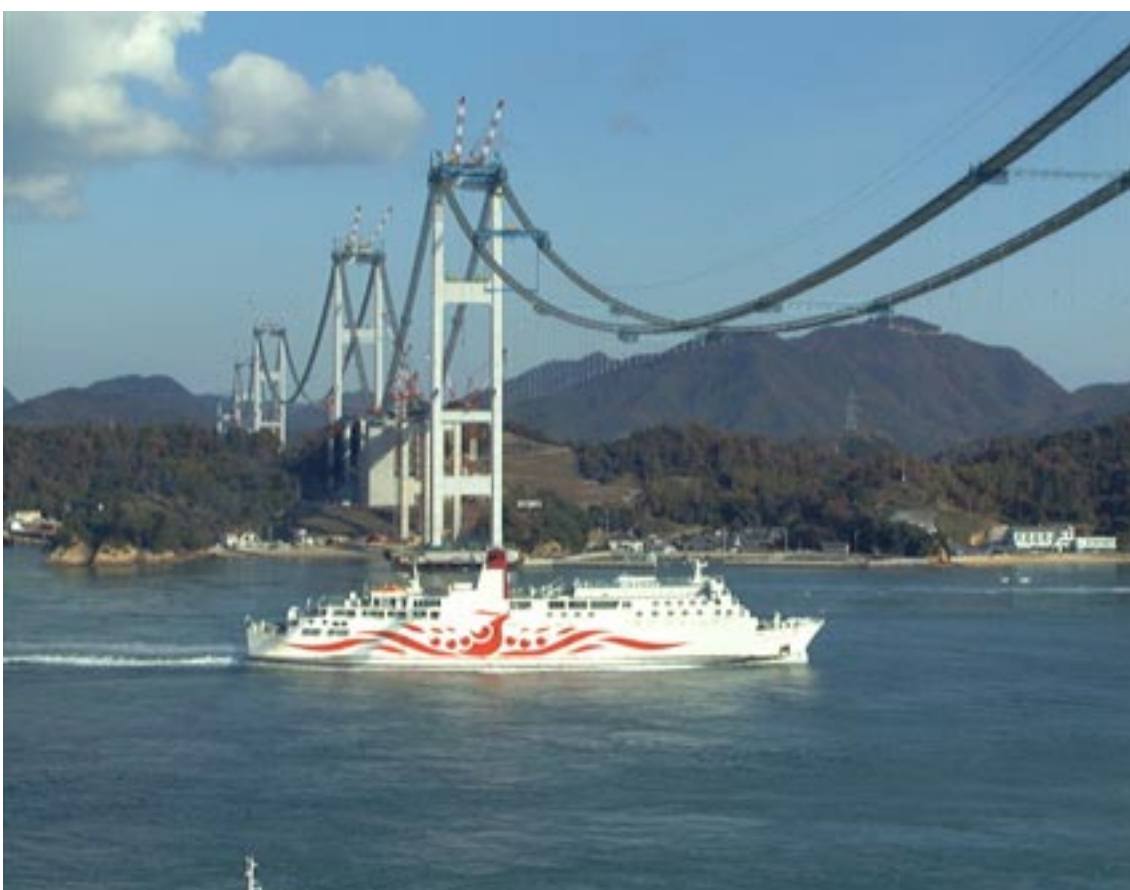
White Sanpou going under the Bridge in construction
